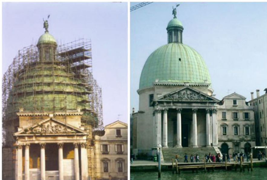
Fig. 2 Architecture that mimics 3-D cellular architecture and tissue repair. The San Simeon Piccolo Dome in Venice, Italy. Each of the metal rods has a diameter of \sim 4 cm, 500 times smaller than the size of the dome with a diameter of \sim 20 m. Each rod also serves as a construction scaffold for building or repairing the dome that is truly embodied in three dimensions ( left panel ). When the repair and construction is completed, the scaffold is removed as shown ( right panel )
